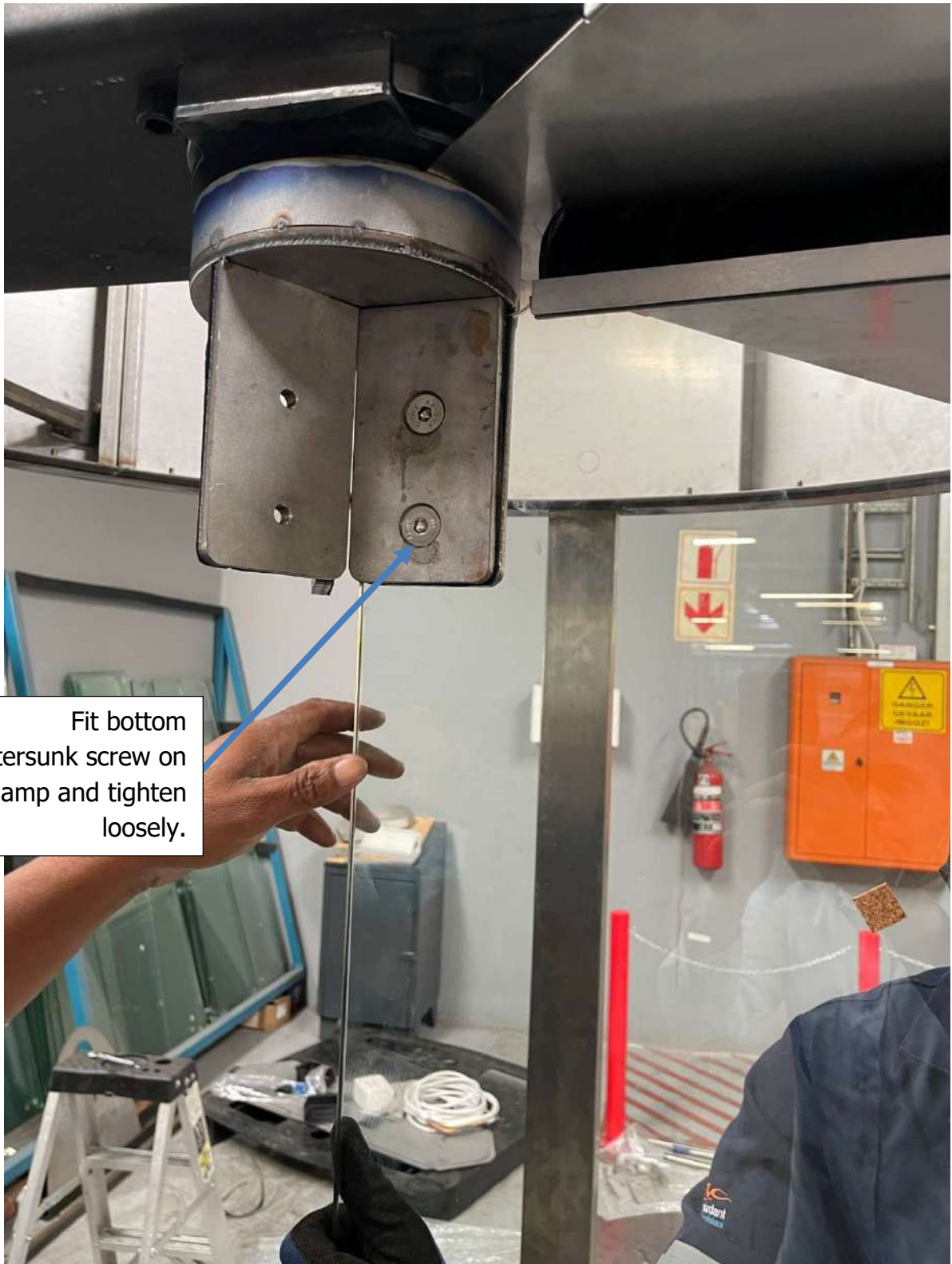
Figure 87: Top glass clamp and screw 2
