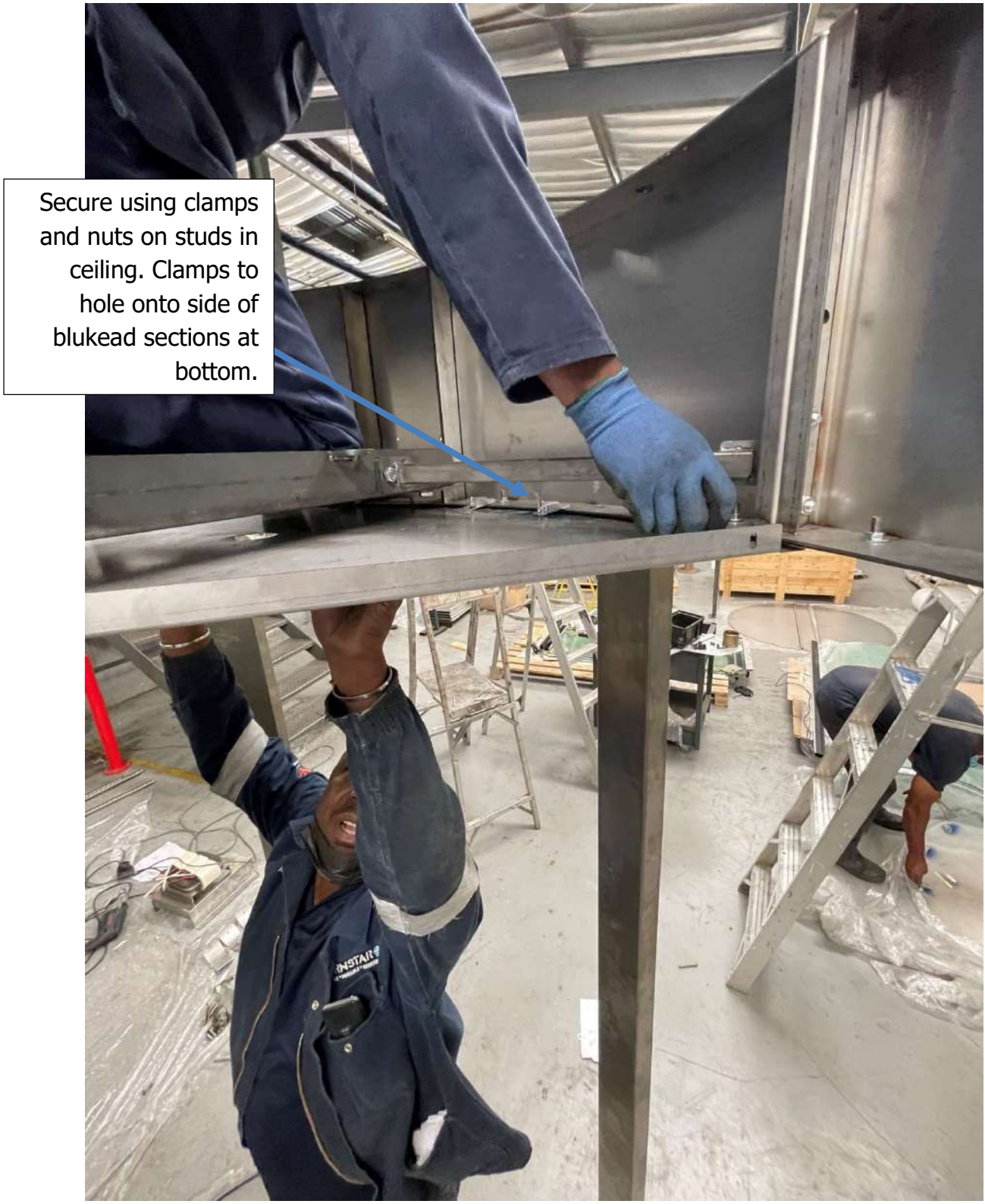
Figure 68: Installing Ceiling plates 2
