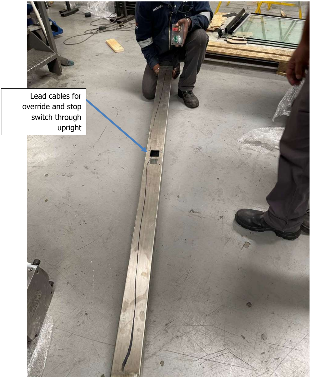
Figure 24: Lead cables through upright
