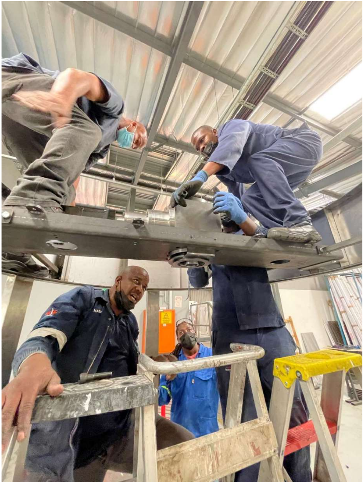
Figure 63: Lifting motor onto center channel 3
