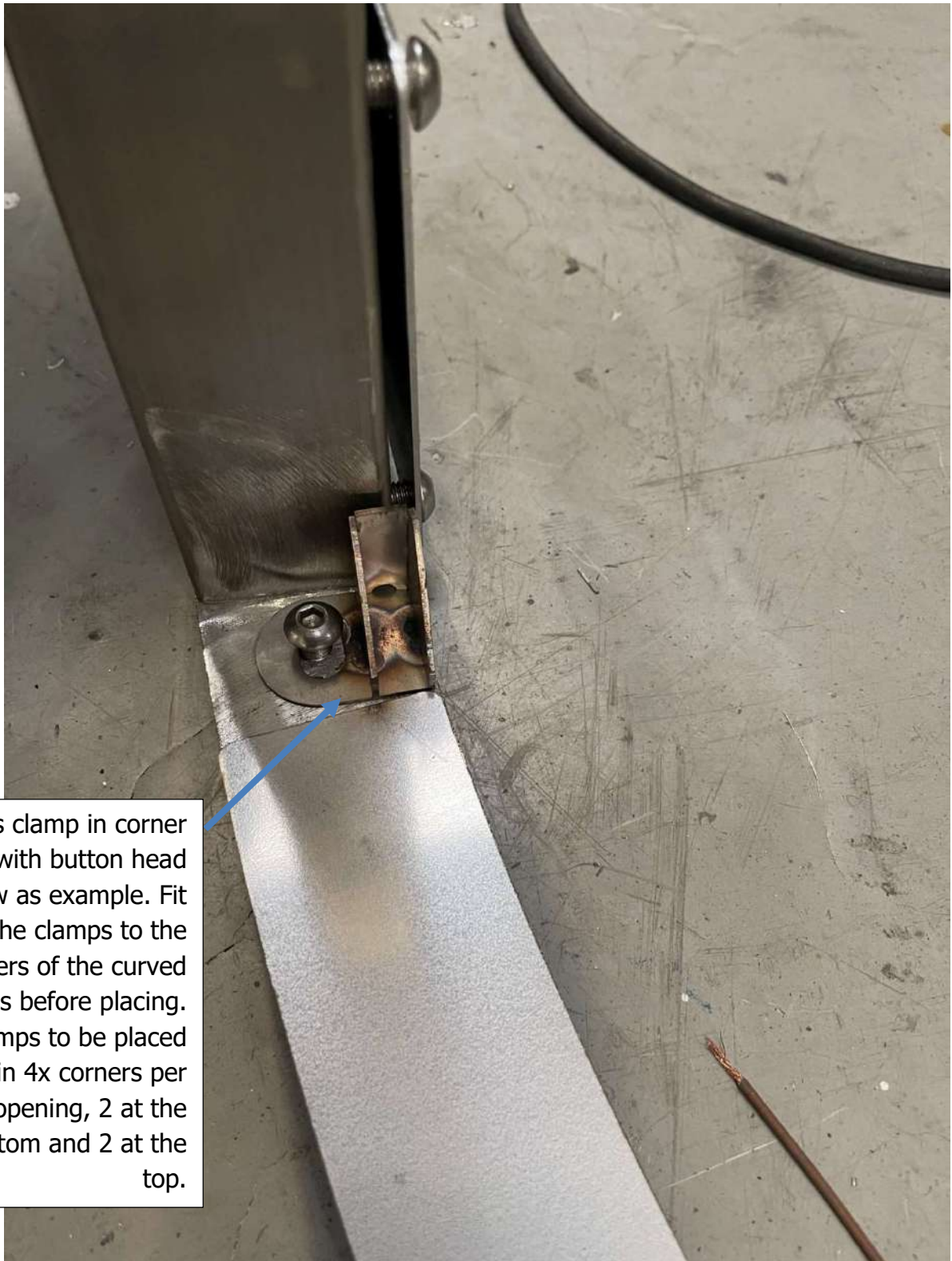
Figure 104: Glass clamps in corners
