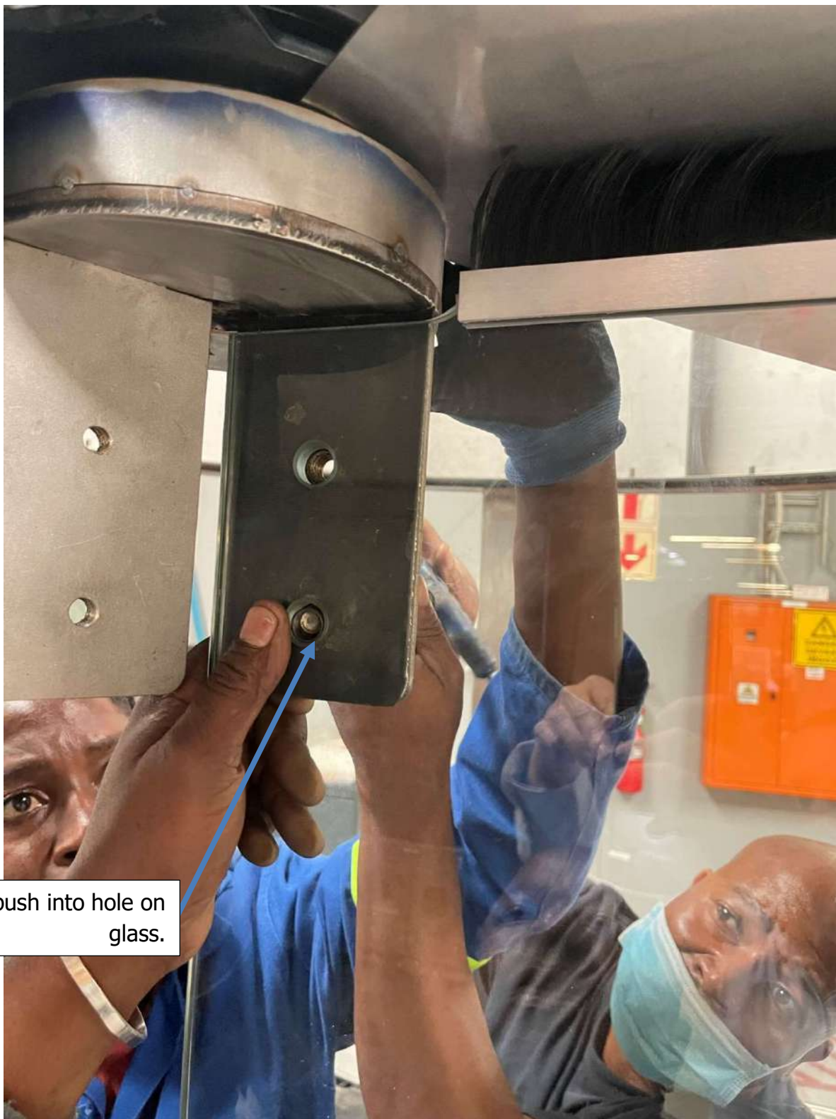
Figure 83: Plastic bush for glass holes 2
