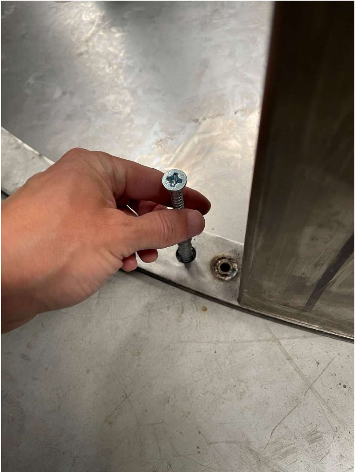
Figure 59: Bolt down the halve outer drum 2
