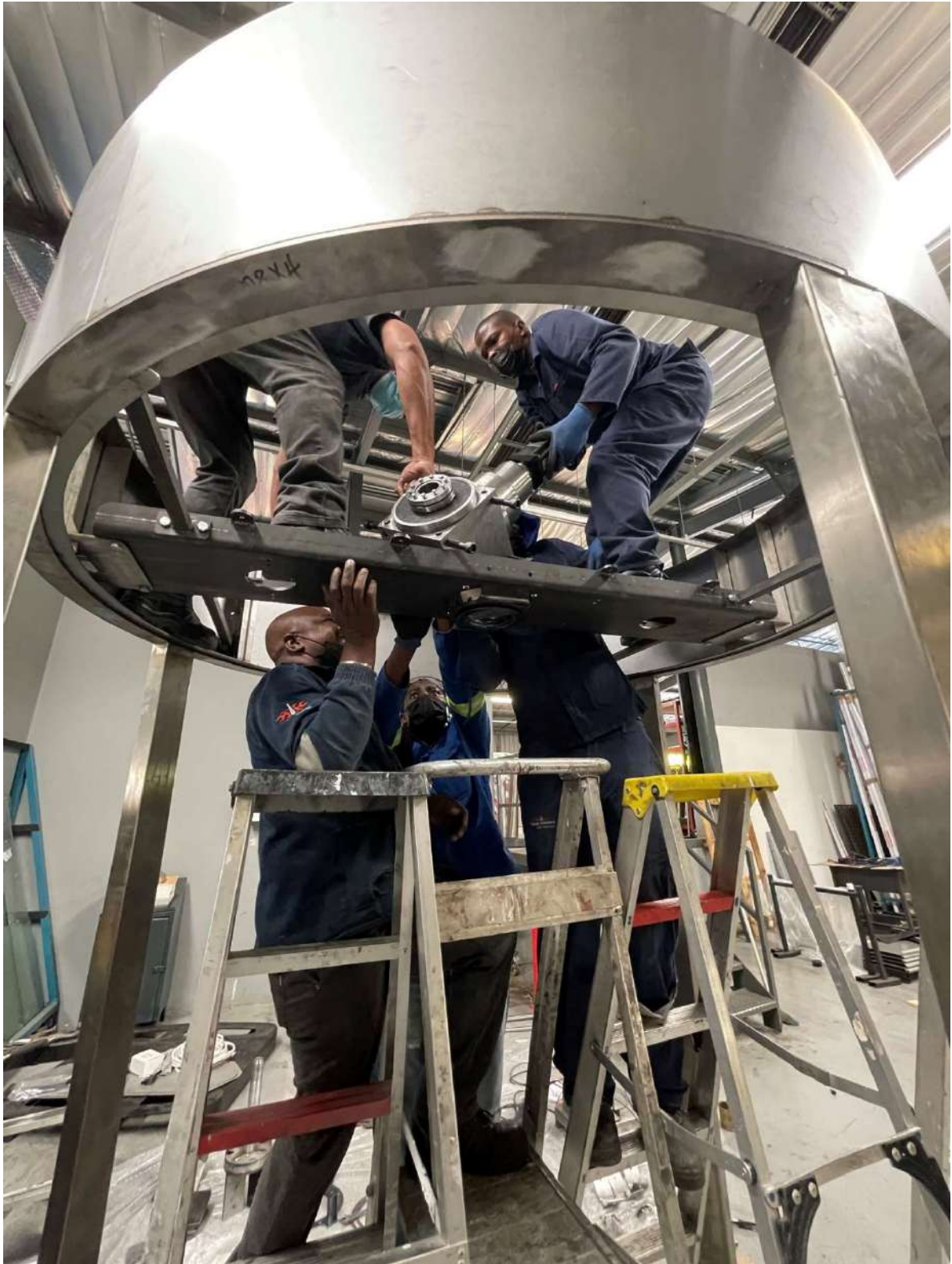
Figure 62: Lifting motor onto center channel 2
