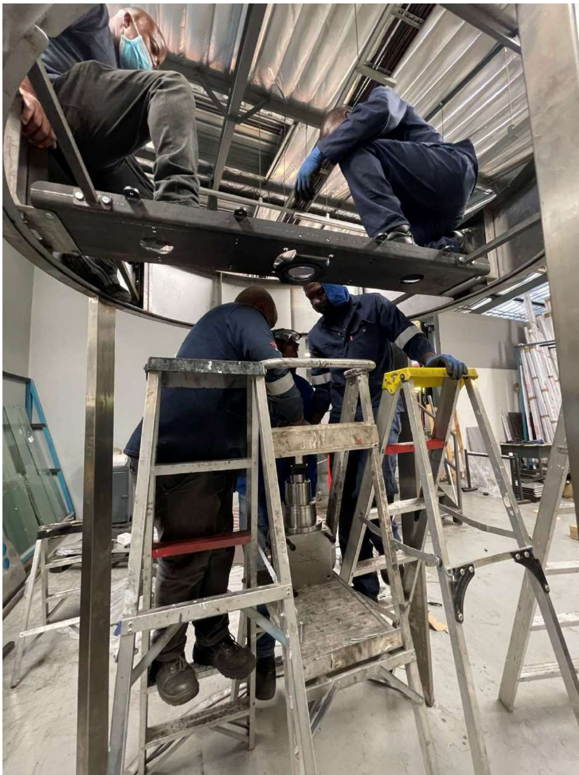
Figure 61: Lifting motor onto center channel
