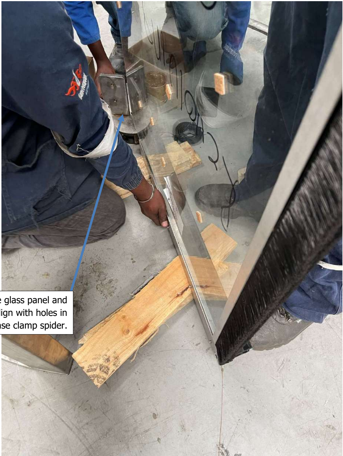
Figure 77: Place glass panel
