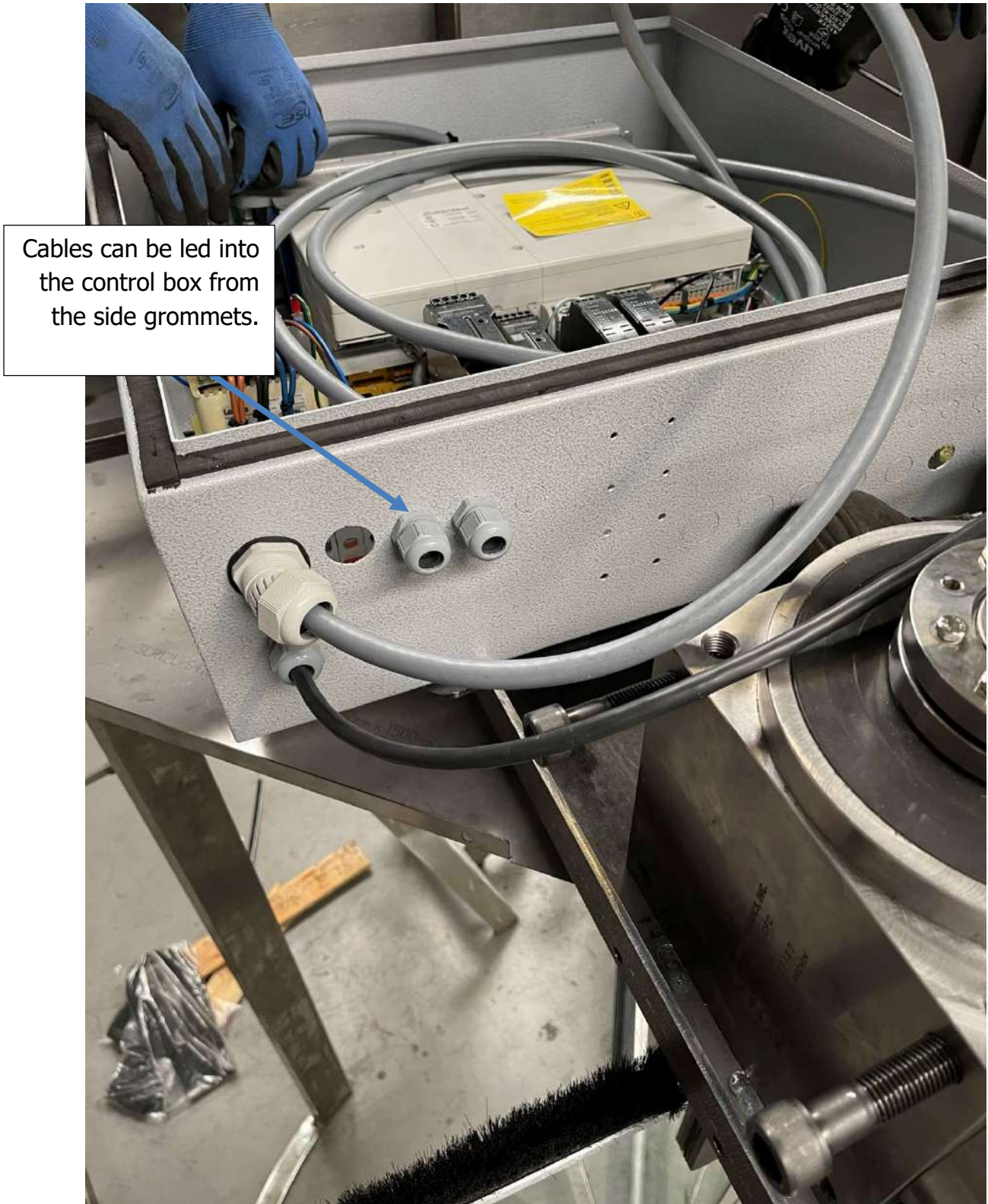
Figure 115: Cables to control box
