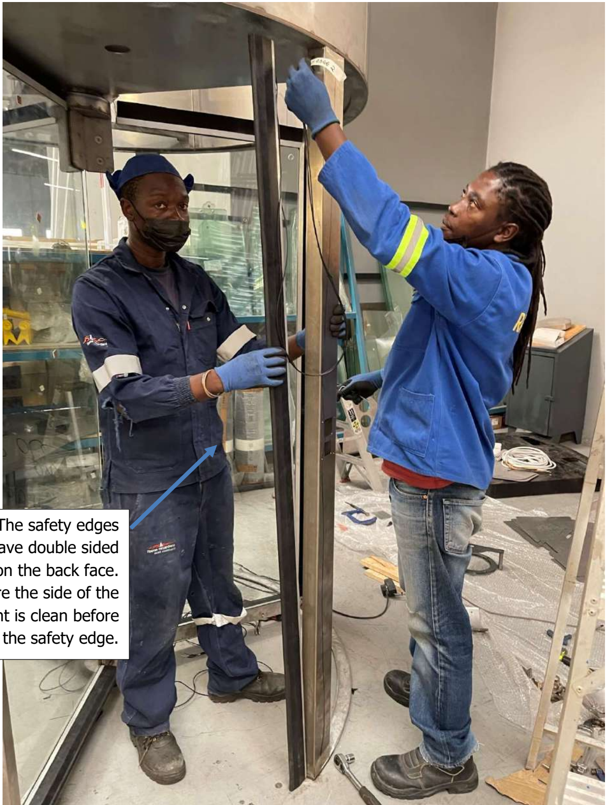
Figure 107: Safety edges on uprights 2
