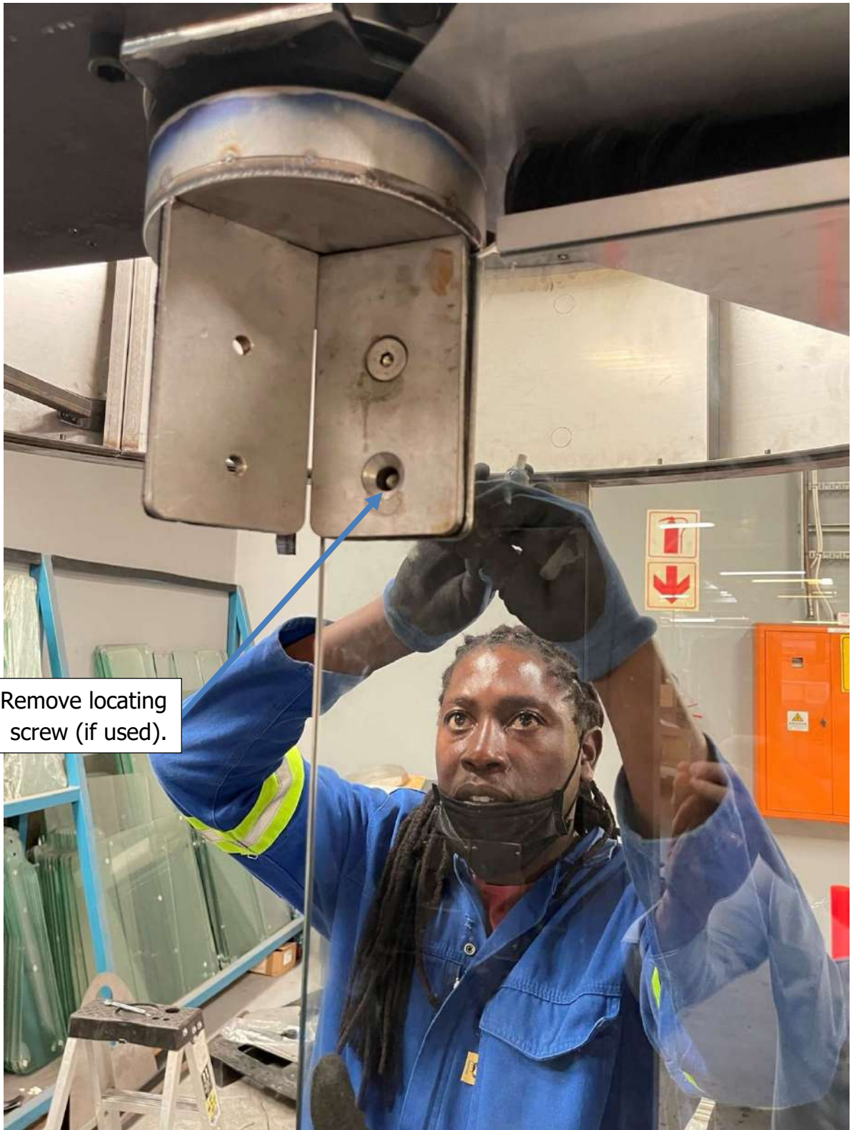
Figure 86: Remove locating screw
