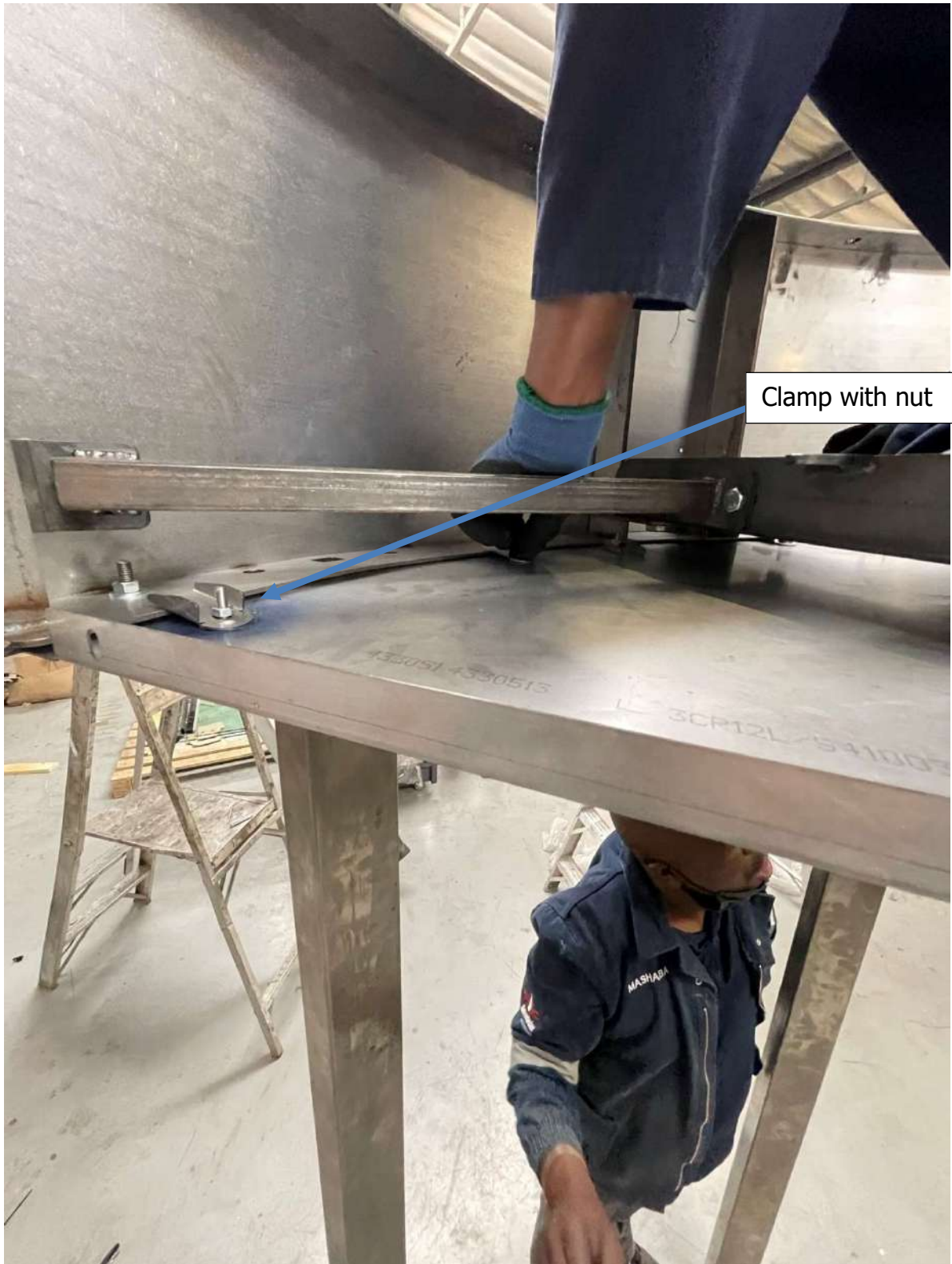
Figure 69: Installing Ceiling plates 3
