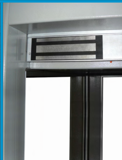
RECESSED 500KG MONITORED MAGNETIC LOCK
