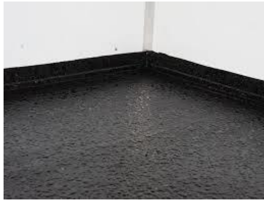
Figure u: Rubberised floor
