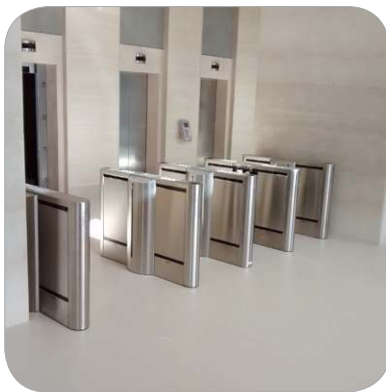
Commercial Building - Brazil
