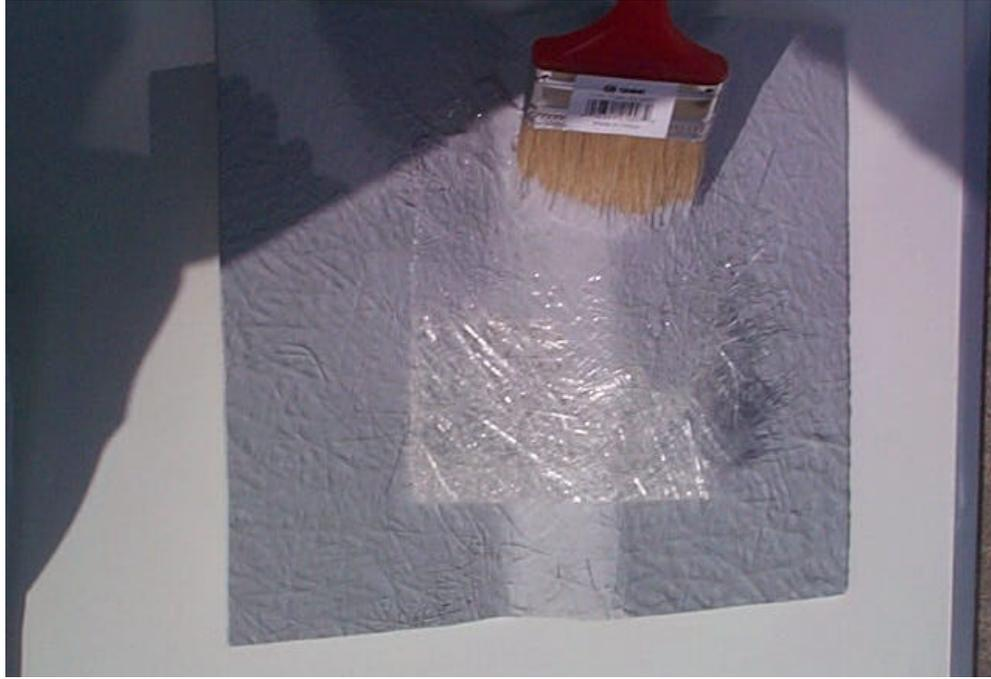
**Step #5:** Let the resin cure for 2 hours at room temperature. Remove the tape from the outside surface. Mix the gray putty supplied in the repair kit with a 1% ratio of catalyst. Apply the putty with a spreader to the outside surface to smooth over the repair on the outside.
