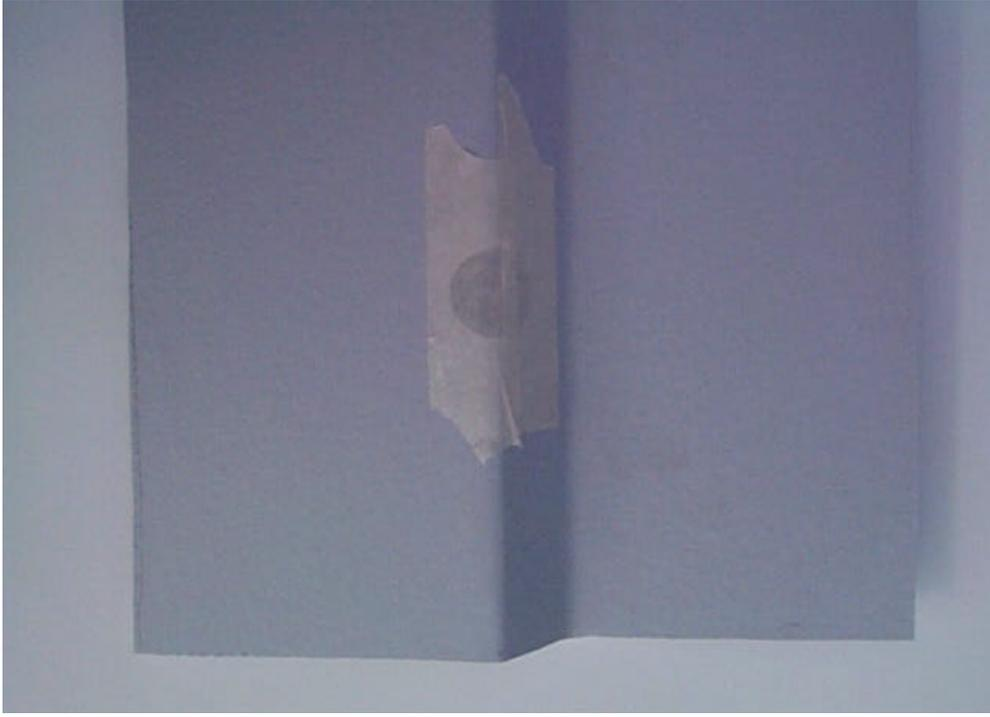
Step #3: Shake the can of resin supplied in the repair kit well. Cut a piece of the dry glass cloth 3" larger than the hole or the area of the repair.
