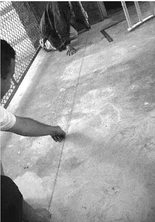
Figure 3.1 - Locating and marking the centerline of the turnstile.
