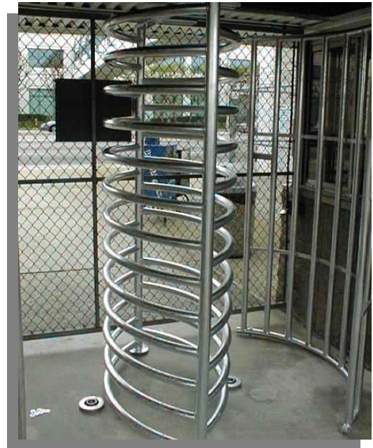
Figure 3.10 - OV section anchored and level. Picture viewed from the outside or unsecured side of the turnstile.
