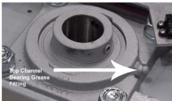
Figure 4.5 – Lubricating the top bearing and top channel
