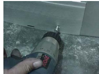
Figure A.8 - Securing the yoke sections to the aluminum yoke mounting channels.
