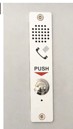
EXTERNAL SIDE PUSHBUTTON, TRAFFIC LIGHTS & INTERCOM
