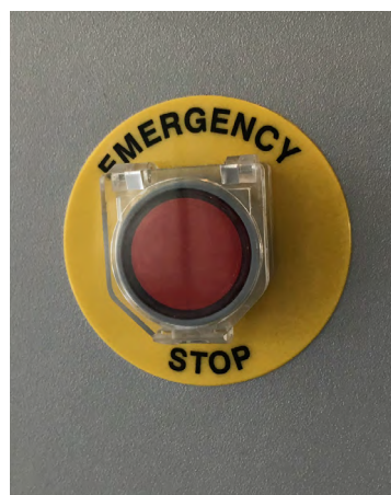
INTERNAL EMERGENCY PUSHBUTTON
